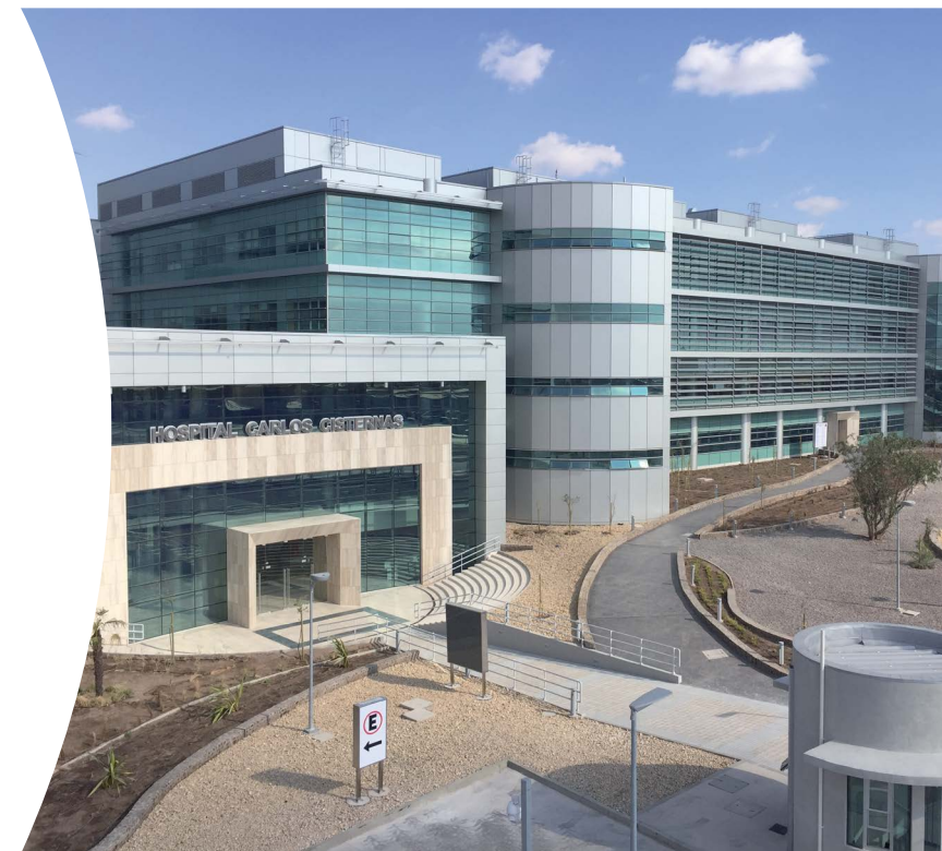
Hospital Carlos Cisternas, Calama (Chile)
